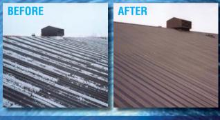
METAL-KOTE colour matched to original plastic coated profile metal roofs. which were flaking and peeling.
